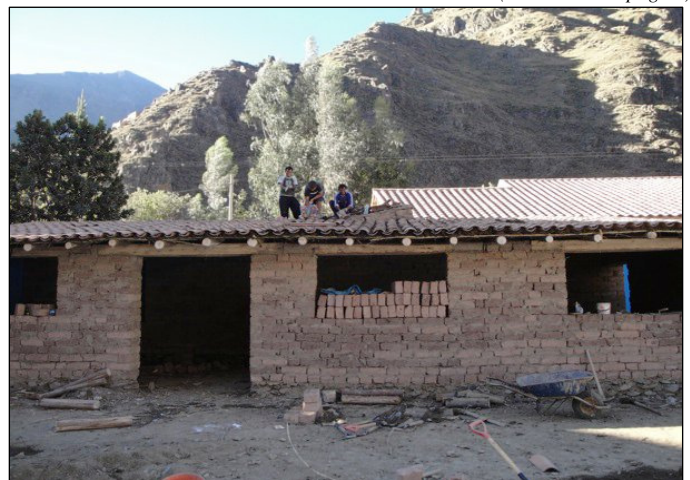
The cafeteria that we helped build, almost finished. (Ollantaytambo, Peru)
